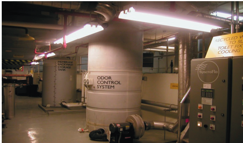
Figure 2. Membrane bioreactor in basement of The Solaire
