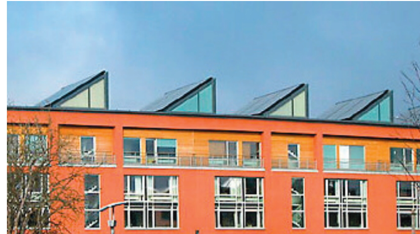
Figure 2.4 Capture of renewable energy by roof solar panels provides heating of water
