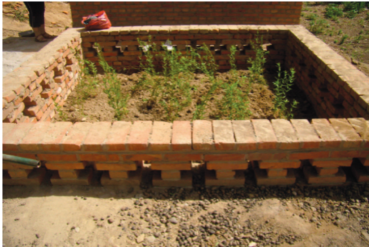
Fig. 6 Biofilter removing odor
