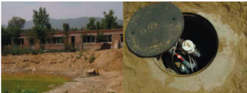
Fig. 4 Northern housing rooms and a collecting tank under construction
