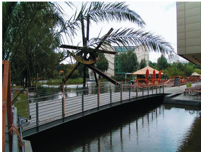
Figure 15. Europes largest stormwater management project at Potsdamer Platz combines green roofs, rainwater harvesting and an urban rainwater lake with a total stormwater retention capacity of 4000 m 3 additional to the green roofs
