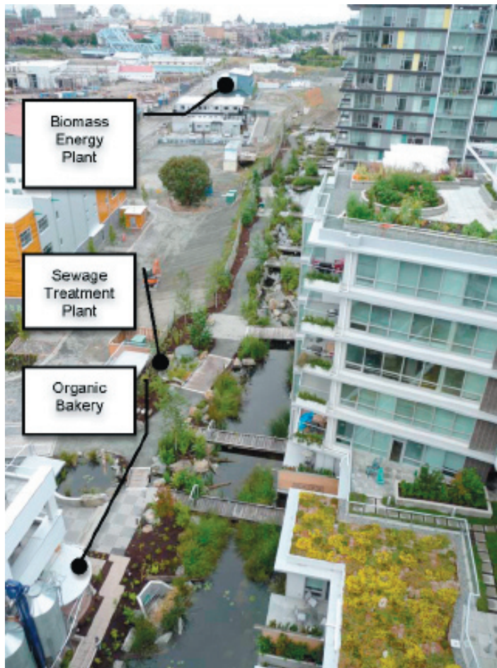
Figure 5. Docksider Green July 2009 showing central stream, green roofs, on-site sewage treatment plant and biomass plant (blue building) in the background (Aqua-Tex photo).
