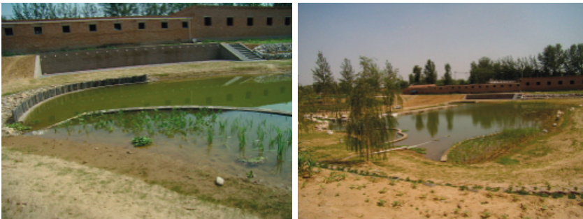
Fig. 13 Rainwater harvesting system and ecological lake
