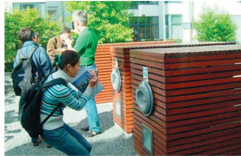
Figure 2.5 Source level separation and disposal of solid wastes into the vacuum conveyance system
