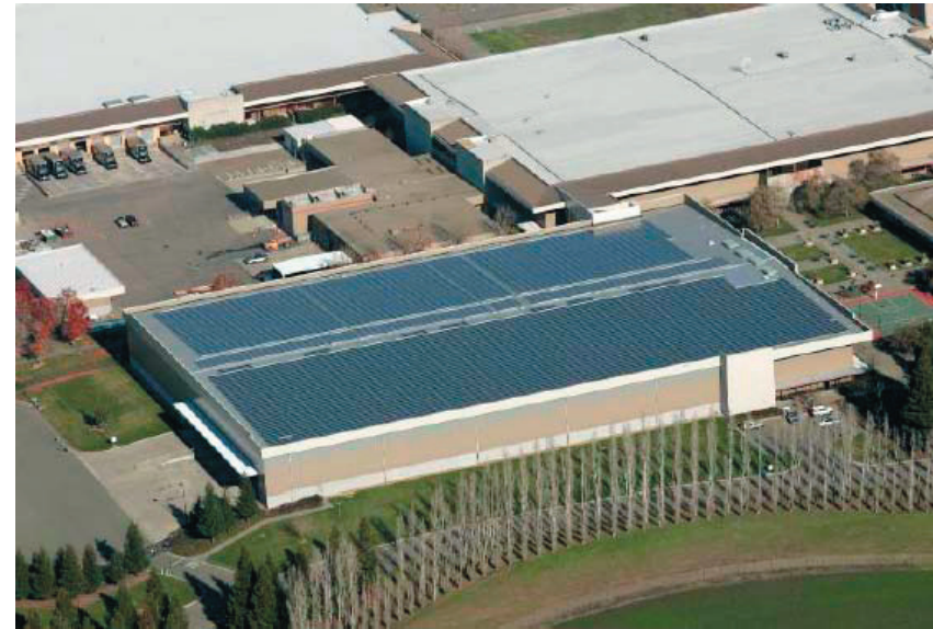
Figure 2.37 Existing solar panels placed on building in 2006. (Sonoma Mountain Village 2008)
