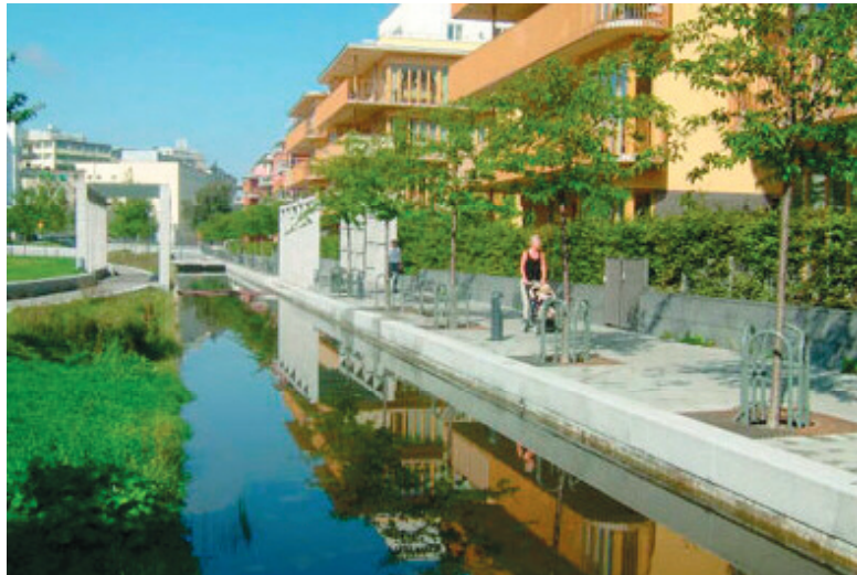
Figure 2.3 Residential area with the surface stormwater channel
